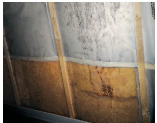
Damage due to the inclusion of damp wood combined with a conventional water vapour retardant.
