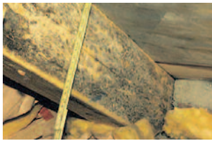
Roof beams infested with mould
