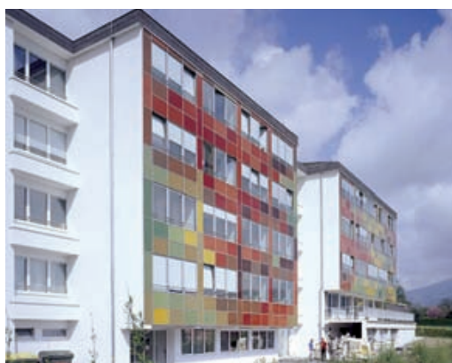
Before and after. Incorporation of the loggias into the building envelope.
