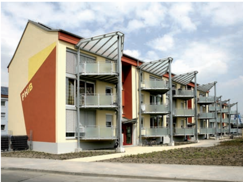
Renovated row of houses with self-supporting balconies (Ludwigshafen, Germany)
