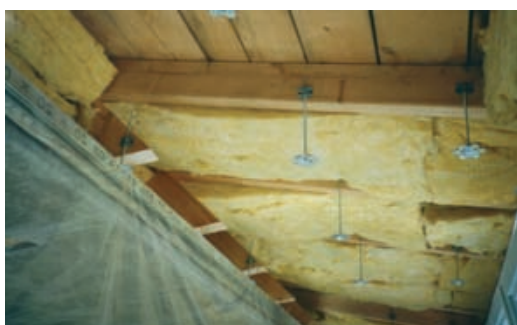
Inside, the roof construction was insulated with 200 mm of ISOVER glass wool between the rafters and the ROSATWIST mounting system.
