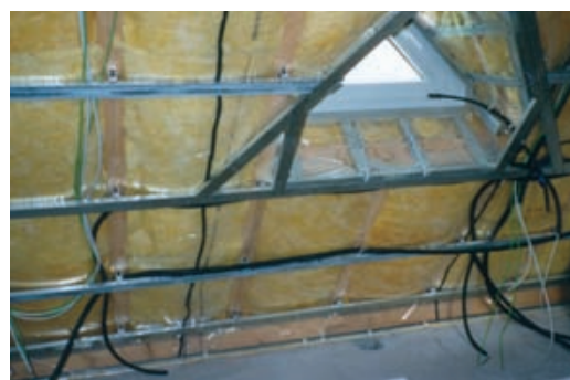
VARIO KM used as vapour barrier and airtight layer. The electrical cables and wires are installed on the room facing side of the membrane which is then insulated with 60 mm glass wool.
