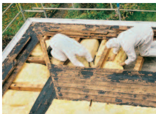
Renovation of a cold flat roof from above, including the waterproofing layer and the roof covering.
