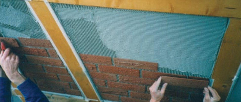
Reconstructed trussed gable. Stone slips were bonded on mineral wool infilling.
