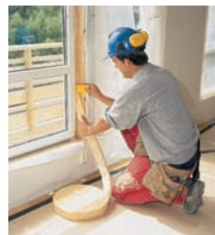
VARIO FS2 provides a perfect, long-lasting seal between window and door frames and adjacent brickwork.
