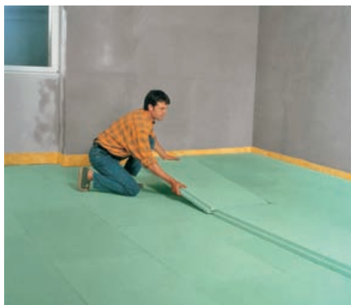
Extruded polystyrene (XPS) insulation boards: double-layered to ensure higher living comfort and lower energy costs.
