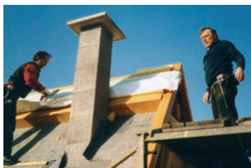
VARIO KM used as vapour barrier and airtight layer. The electrical cables and wires are installed on the room facing side of the membrane which is then insulated with 60 mm glass wool.
