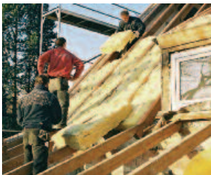
Fitting insulation between fully exposed roof trusses
