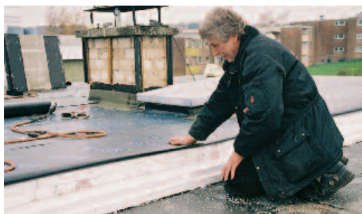
Renovation of a "warm" roof with expanded polystyrene boards
