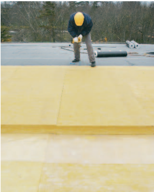
Flat roof with ISOVER glass wool
