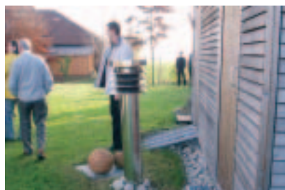
The nose of a passive house: air duct for fresh air supply.
